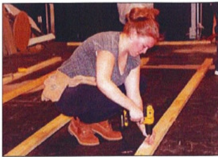
Cardinal Carter student Alyssa Orlando uses a cordless drill to secure a two-by-four to the stage surface at The Bank Theatre to accommodate a new layer of soundproof foam sheathing.
